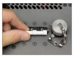
Figure 3.16.2 Switching Circuit Breaker OFF
