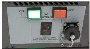
Figure 3.12.2 DC Output "ON" Button is Illuminated
